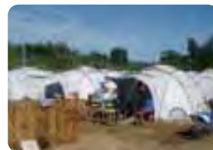
Installing flushing toilets for typhoon victims living in tents (Philippines)
