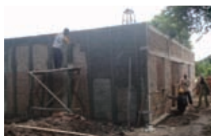
Regional Health Center (Under Construction)
