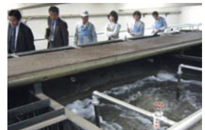
Verification of effectiveness of wastewater treatment facility
